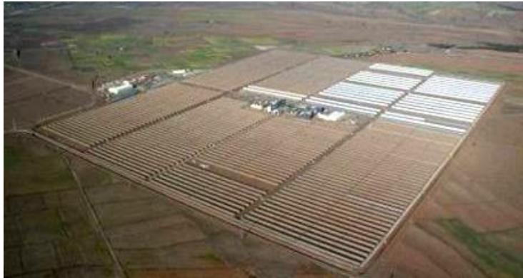
ANDASOL-I plant (Granada, Spain)
