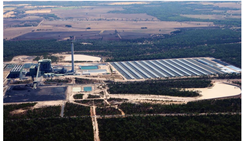
44-MW Kogan Creek Solar Boost in Queensland, Australia
