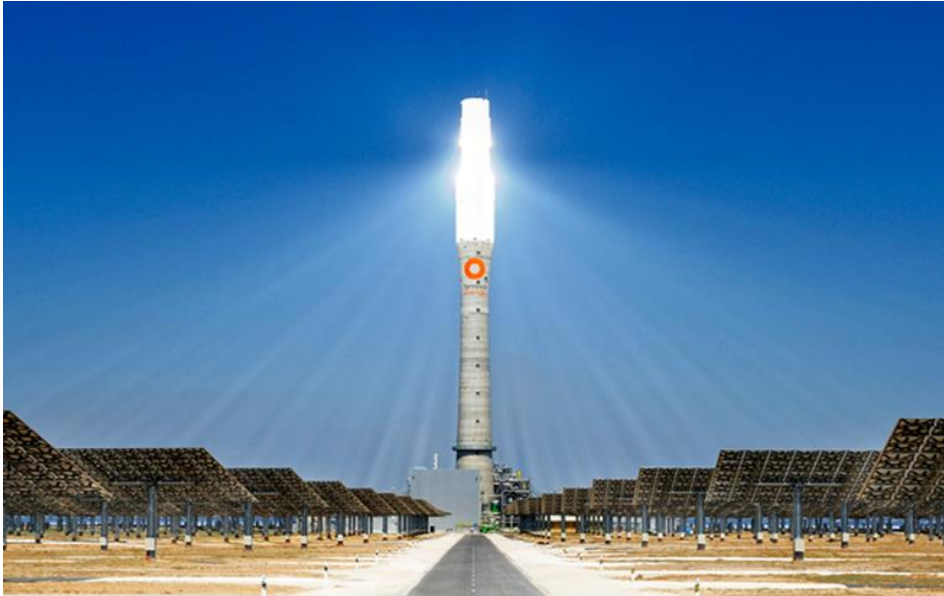
Tower using molten salts GEMASOLAR 17 MWe October 2011 15h thermal storage !! Spain
