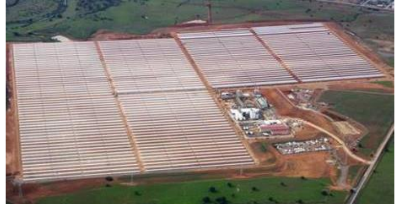
IBERSOL plant (Ciudad Real, Spain)
